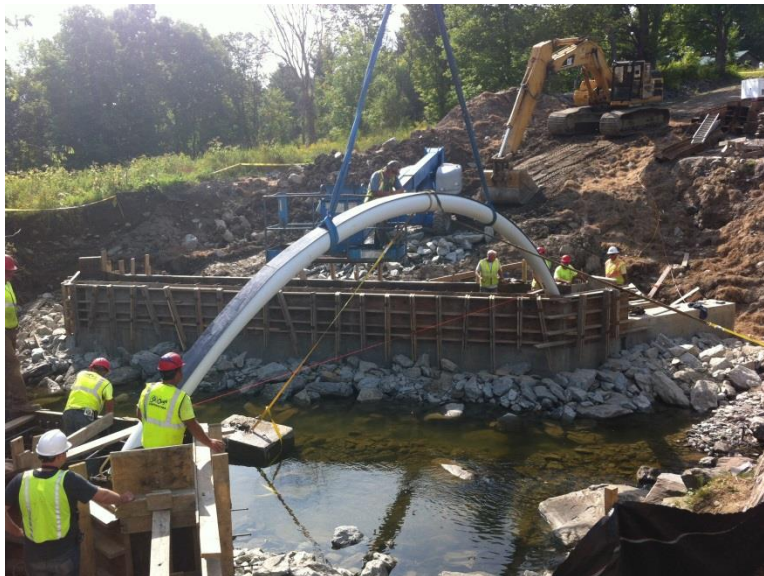
Figure 8 Installation of the first tube (VTrans)
