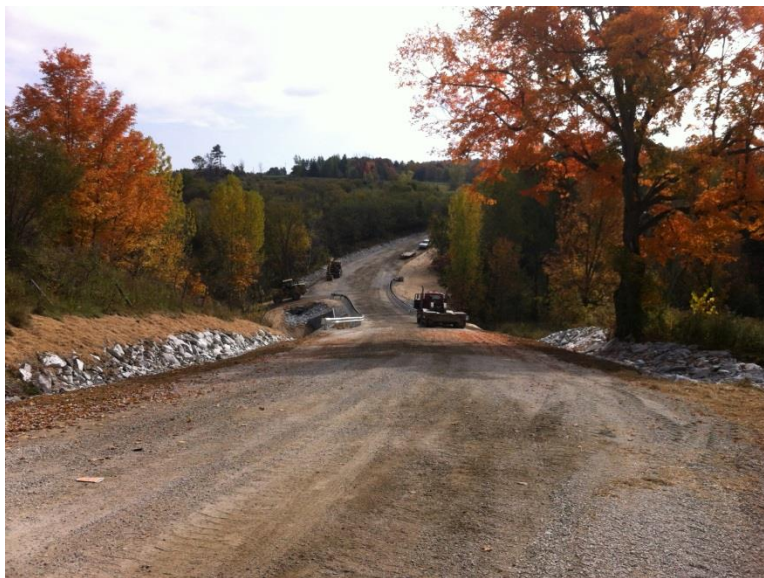
Figure 14 Completed project (VTrans)
