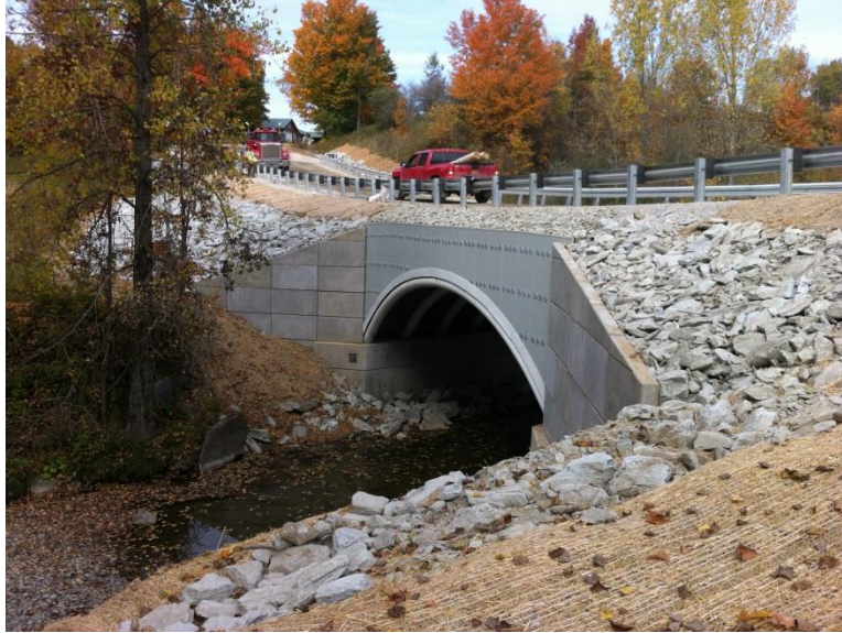
Figure 13 Completed Bridge in a Backpack (VTrans)
