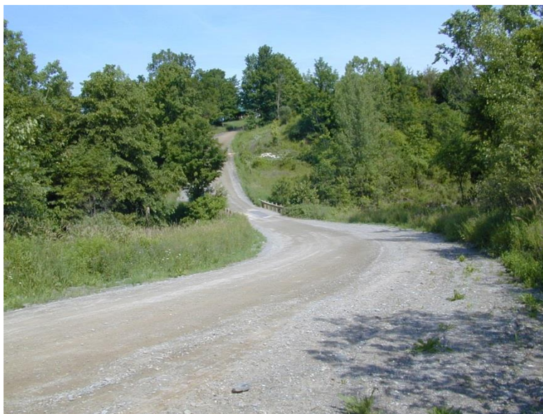
Figure 3 Bridge 48 alignment (VTrans)
