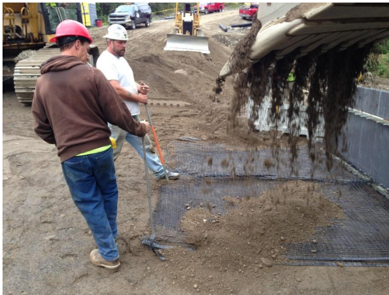
Figure 12 Applying subbase material over geotextile layers (ATI)
