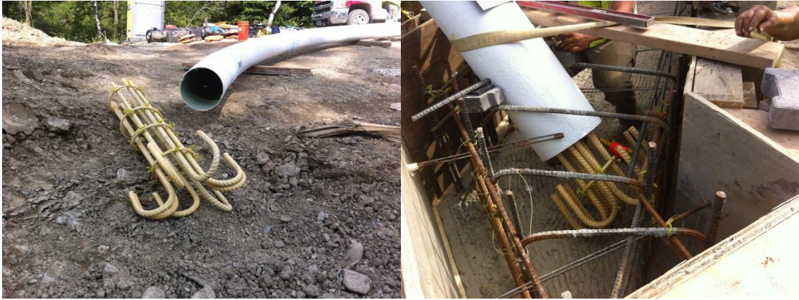
Figure 9 Anchorage reinforcement of the tubes (VTrans)
