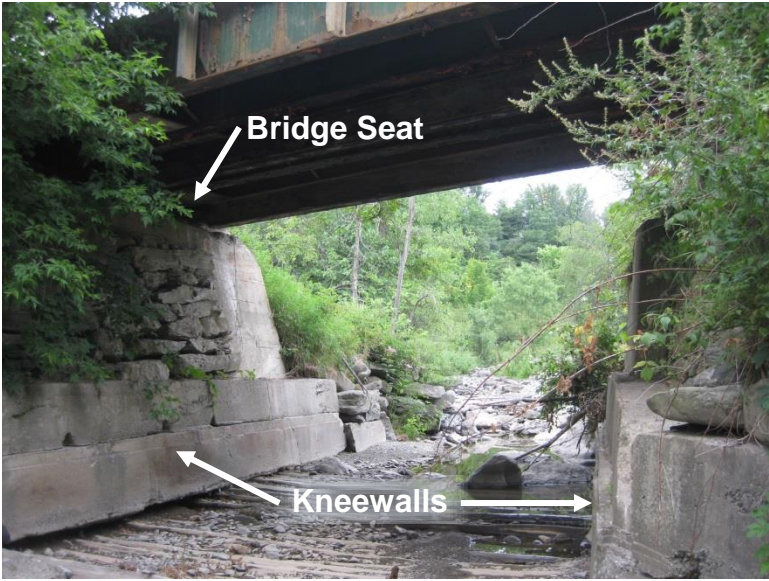
Figure 6 Existing substructure (VTrans)
