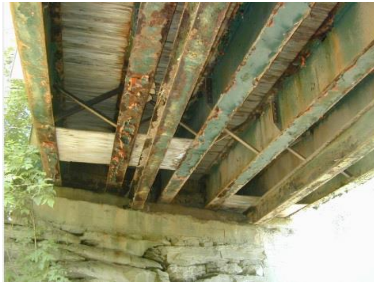
Figure 5 The underside of bridge 48 showing the added beams (VTrans)
