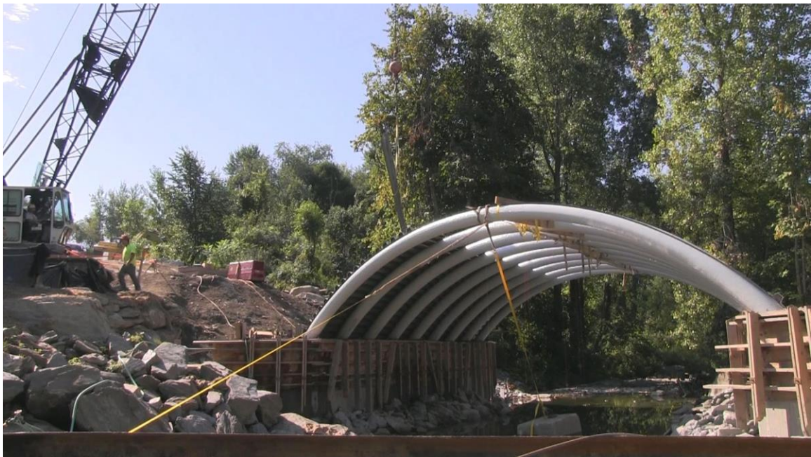
Figure 10 All tubes in place with decking being installed (AP) (18)
