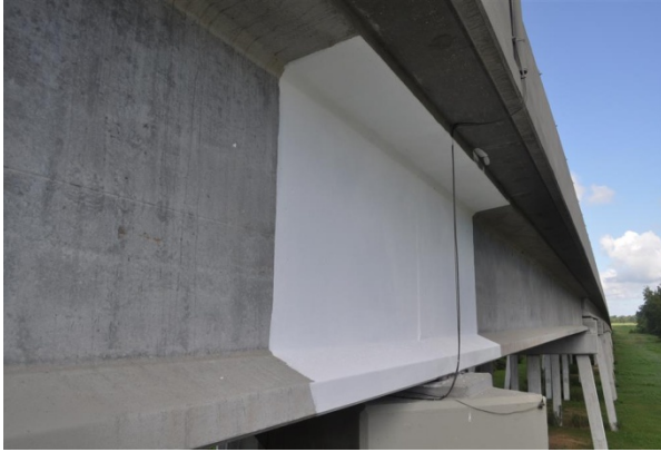
(a) Girder G1 at Bent 24
