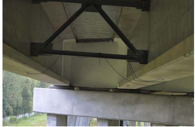
(b) Diaphragm between G1 and G2 at Bent 25
