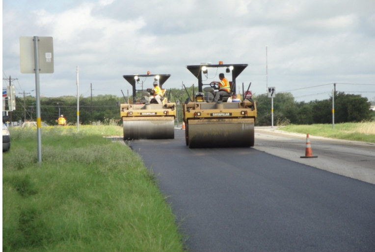
Figure 14. Tandem Roller Compaction (Bryan-Fine SMA).
