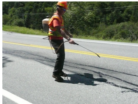
E. Water spraying to cool cracks quicker.
