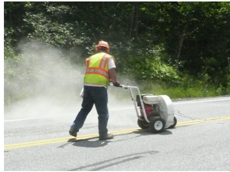
B. Cleaning the crack with a blower.
