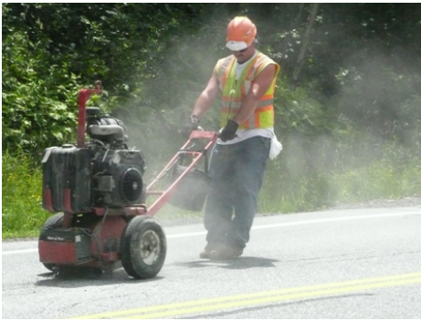
A. Routing the crack.
