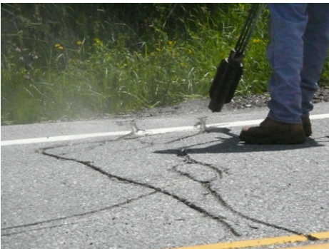
C. Further cleaning with a heat wand.
