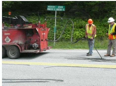
D. Filling of routed cracks with fill material.
