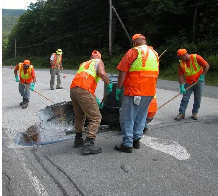
Figure 8 Placement of the second lift.
