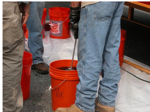
Figure 5 Mixing the Epoxy
