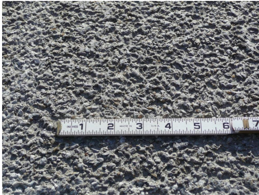
Figure 11 The texture of the SafeLane overlay after a year of service.
