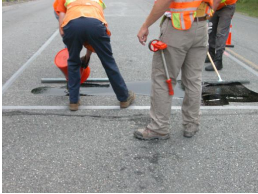
Figure 6 Spreading Epoxy
