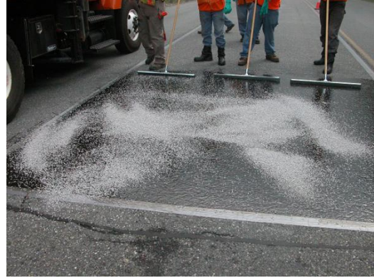
Figure 7 Spreading limestone
