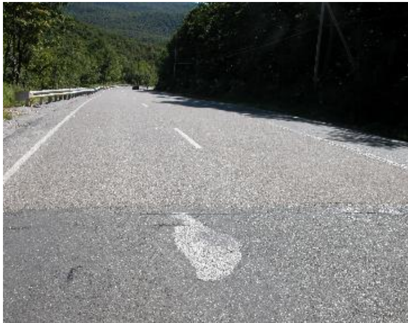
Figure 9 Completed overlay
