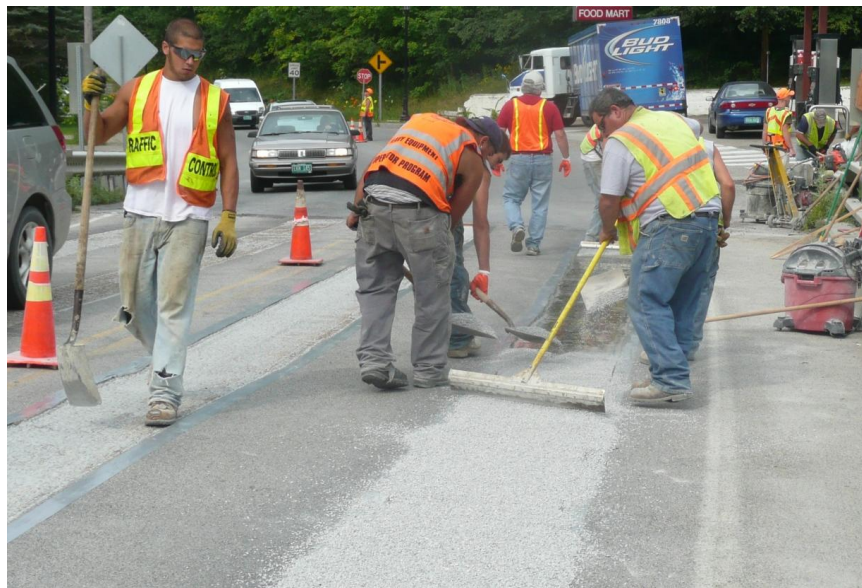
Figure 20 Repairing the wheel paths.
