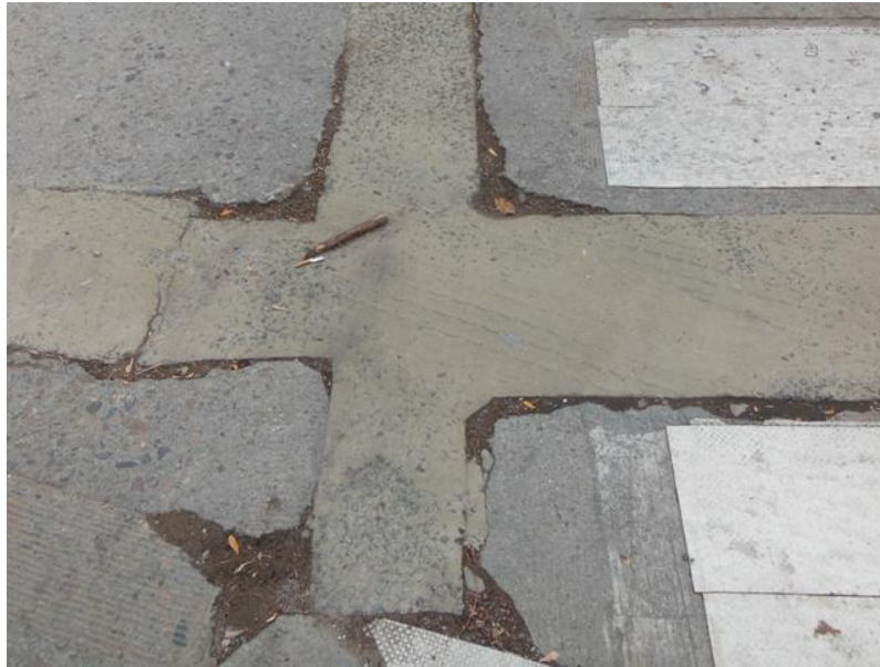
Figure 16 Condition of some repair areas following the fourth winter of service life (2013).
