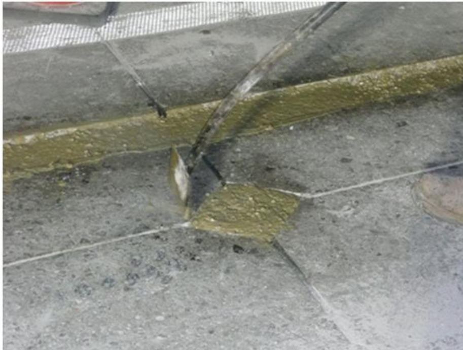
Figure 9 Hot iron used during TechCrete placement for leveling
