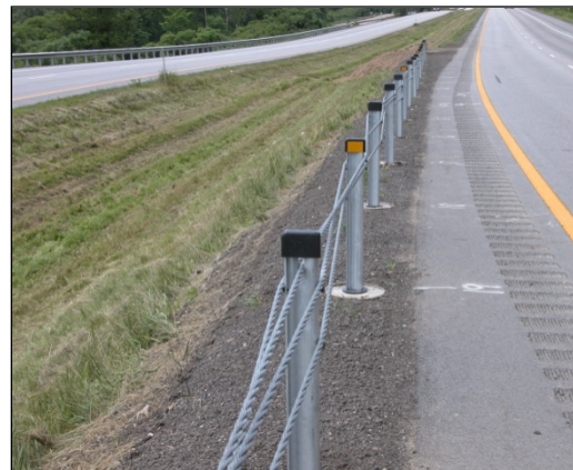
Figure 3: Brifen Wire Rope Fence Showing Interwoven Wire Ropes
