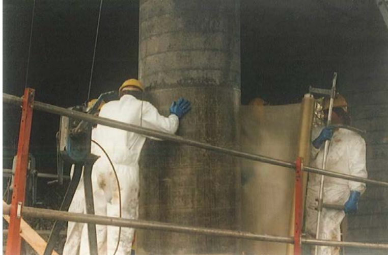
Figure 3: TYFO S Fibrwrap spindle application (1994)
