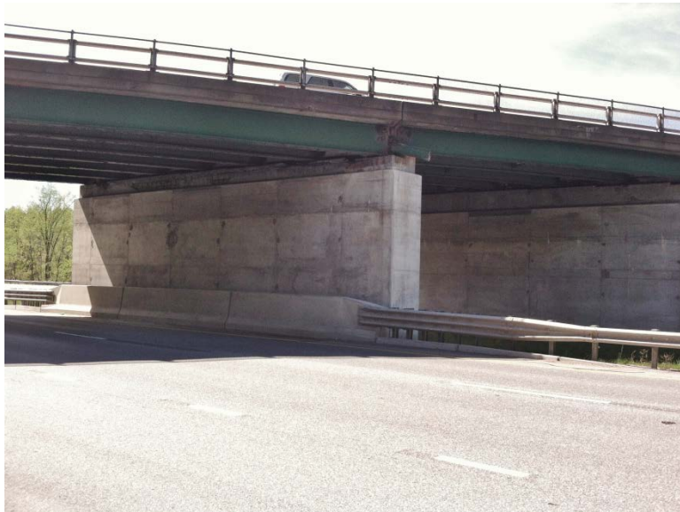
Figure 1 Example of a Mass Concrete Encasement of Pier Columns.
