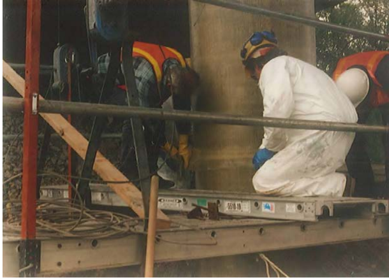
Figure 4 Applying the six inch strip to seal the butt joint (1994).
