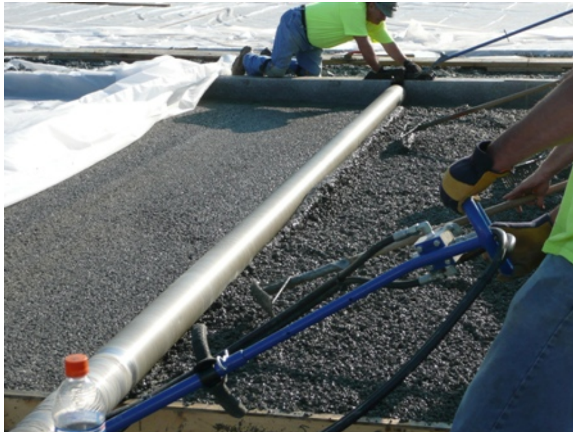
Figure 3. Placement and rolling of porous concrete.
