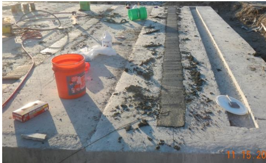
Figure 0.16 Repair material during placement
