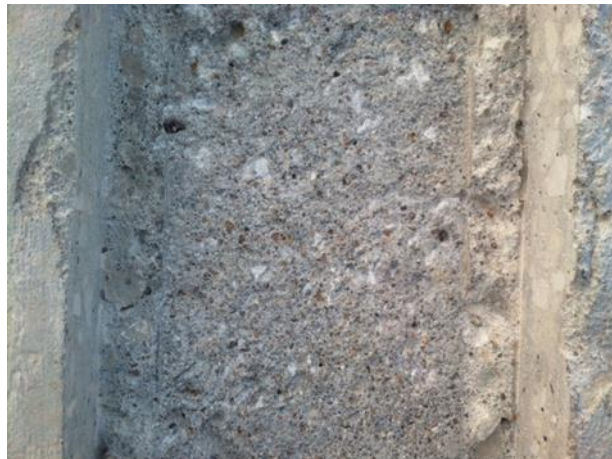
Figure 0.11 Prepared concrete surface
