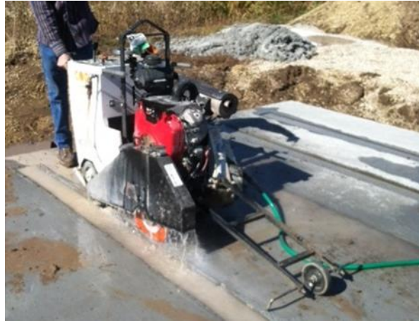
Figure 0.10 Saw cutting of edges
