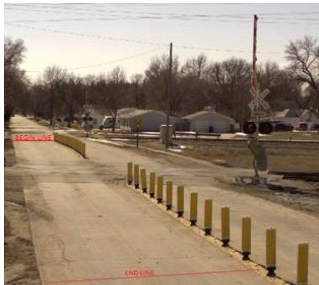
Figure 3.1 Basic area-of-interest at an HRGC (sample: Fremont HRGC)
