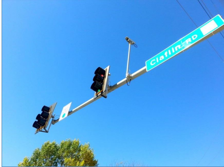
Figure 0.12 Signal backplates at treatment site – 2 before adding reflective tape
