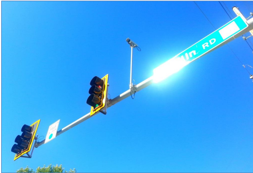
Figure 0.15 Signal backplates at Treatment site – 2 (Denison/Claflin) after adding reflective tape
