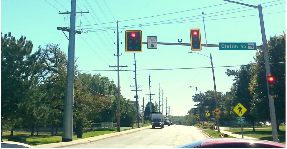
Figure 0.16 Signal backplates at Treatment site – 2 (Denison/Clafin) after adding reflective tape
