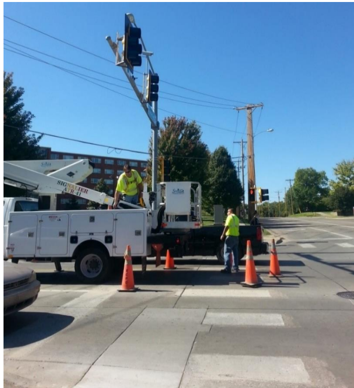
Figure 0.13 Installation of reflective tape – treatment site – 2
