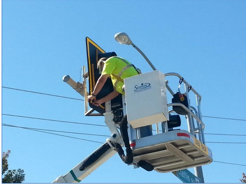
Figure 0.14 Treatment site – 2: Denison Ave. at Claflin Rd.
