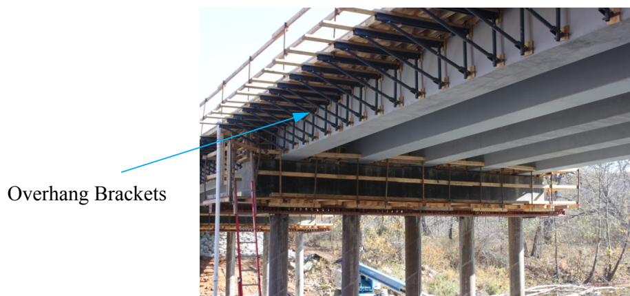
Figure 3-4 Construction of B0439 Superstructure
