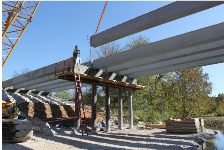
Figure 3-3 Installation of B0439 HCBs on the piers
