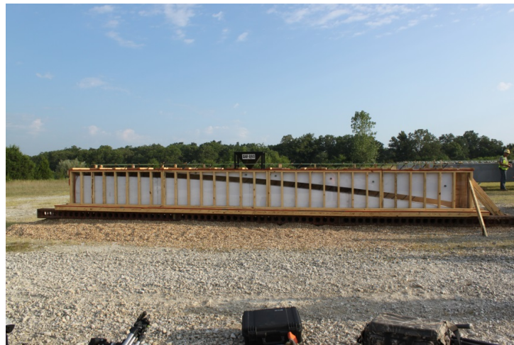
Figure 4-6 Mock-Up Beam Simulates HCB of B0439 (before pour)
