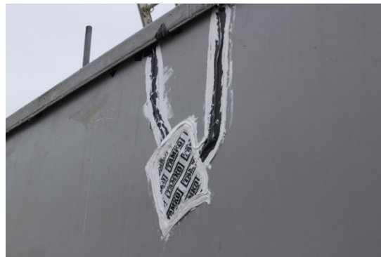
Figure 3-18 FRP Strain Gauge Placement, Final Protection of Gauges and Wiring
