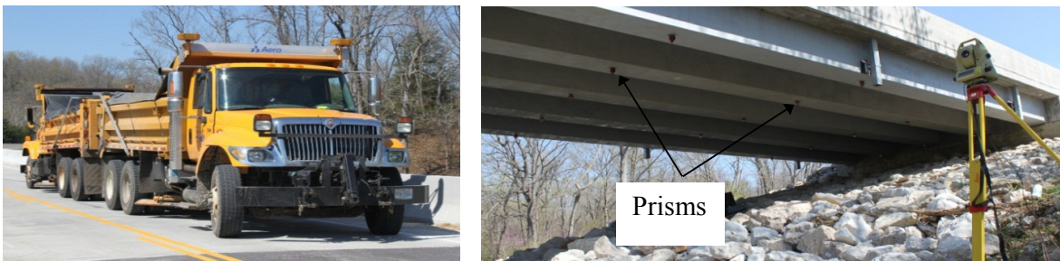
Figure 5-1 Load Test of Bridge B0439; MoDOT Trucks (Left Image); Total station and prisms (Right Image)
