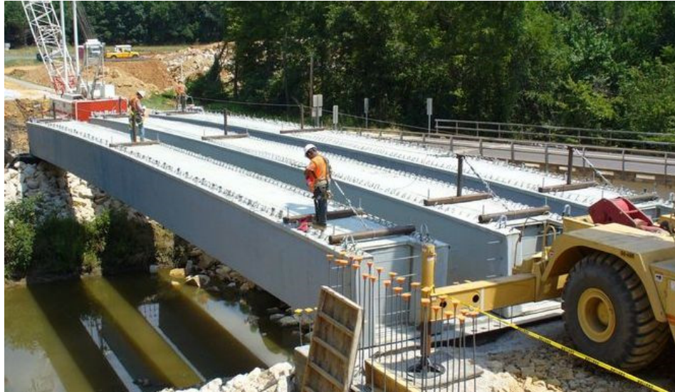
Figure 3-10 Erection of B0410 Double-Web HCBs
