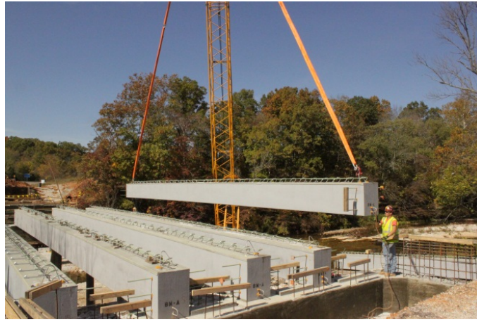
Figure 2-6 Erection Process of B0439 HCB
