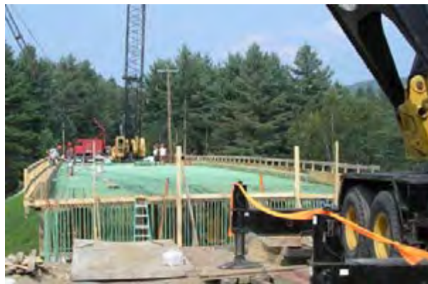
Figure 7-3: Forms and Reinforcement Bars at the Middlesex Bridge
