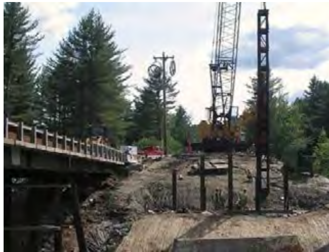
Figure 7-1: Pile Driving at the Middlesex Bridge
