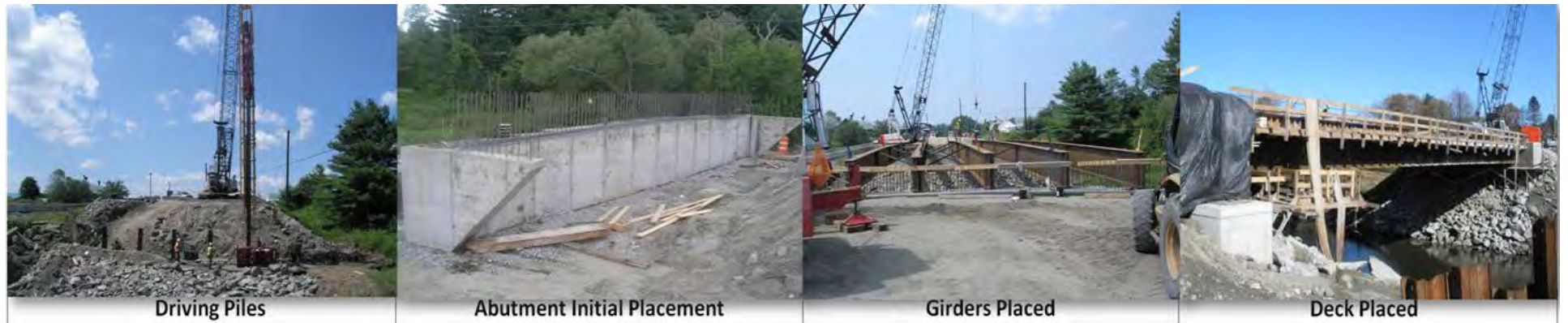
Figure C-0-5: East Montpelier Bridge Construction
