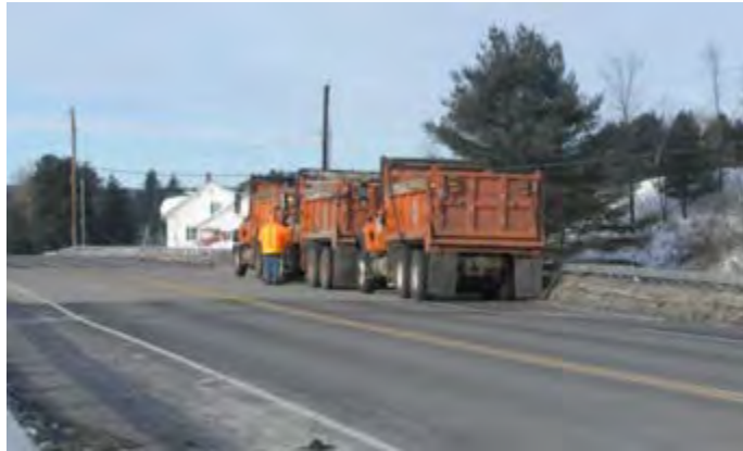
Figure 5-10: East Montpelier Load Testing (Longitudinal Arrangement of Trucks)
