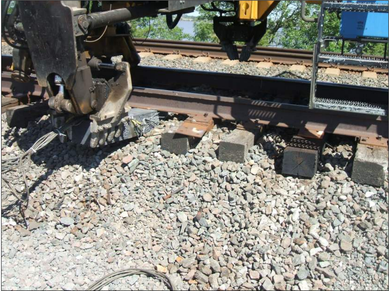
Figure 20. Maximum bending during tie installation.
