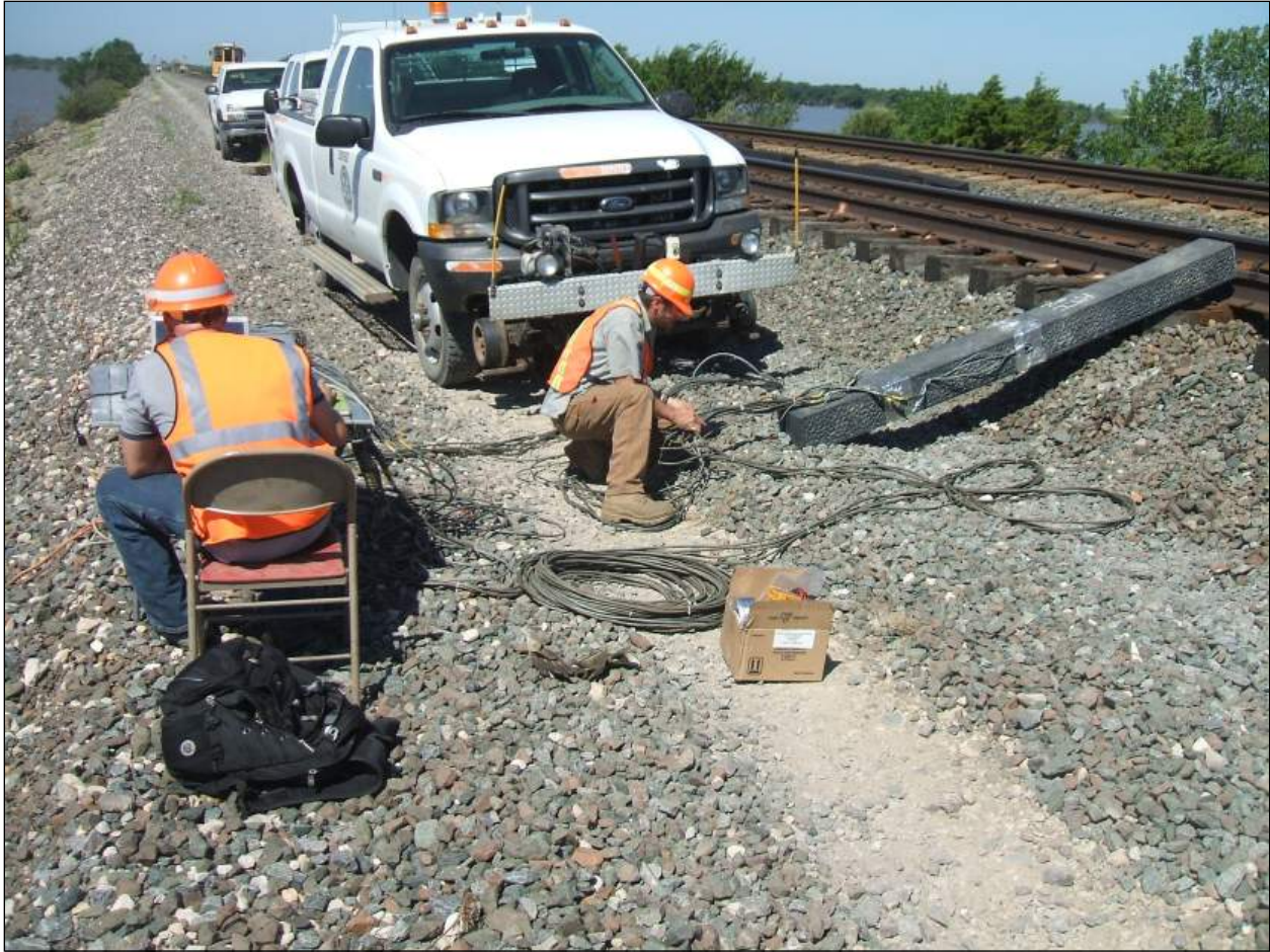
Figure 18. Instrumented tie being prepared for installation at BNSF site.
