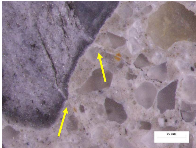
Figure 4.5. A magnified view of the polished cross section in Core C8-1. Note the intersecting fractures that originate in a reactive coarse aggregate particle, extend outward into the surrounding paste structure, and are partially filled with gray, subtranslucent to opaque ASR gel (yellow arrows).
