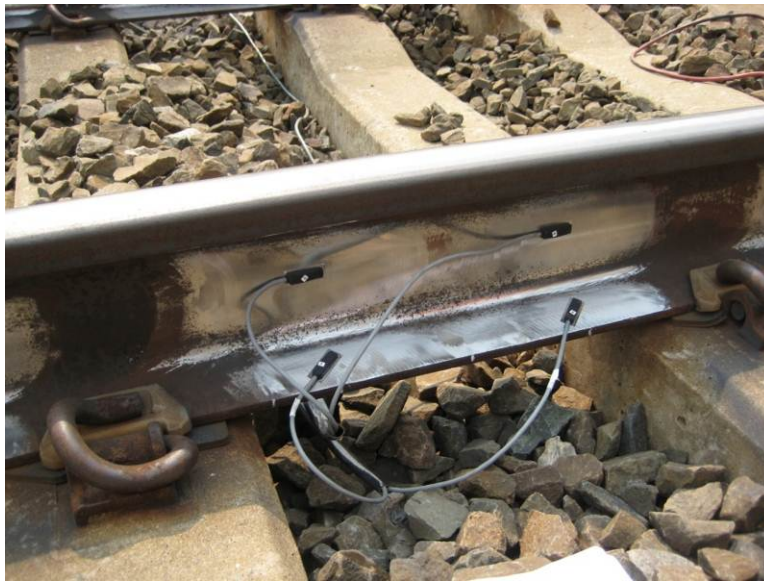
Figure 6.3. Vertical and lateral wheel-rail load strain gages.
