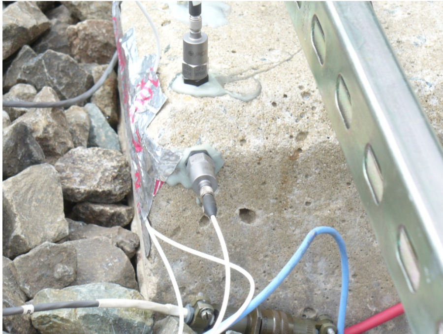
Figure 6.7. Three accelerometers mounted to one end of the tie.
