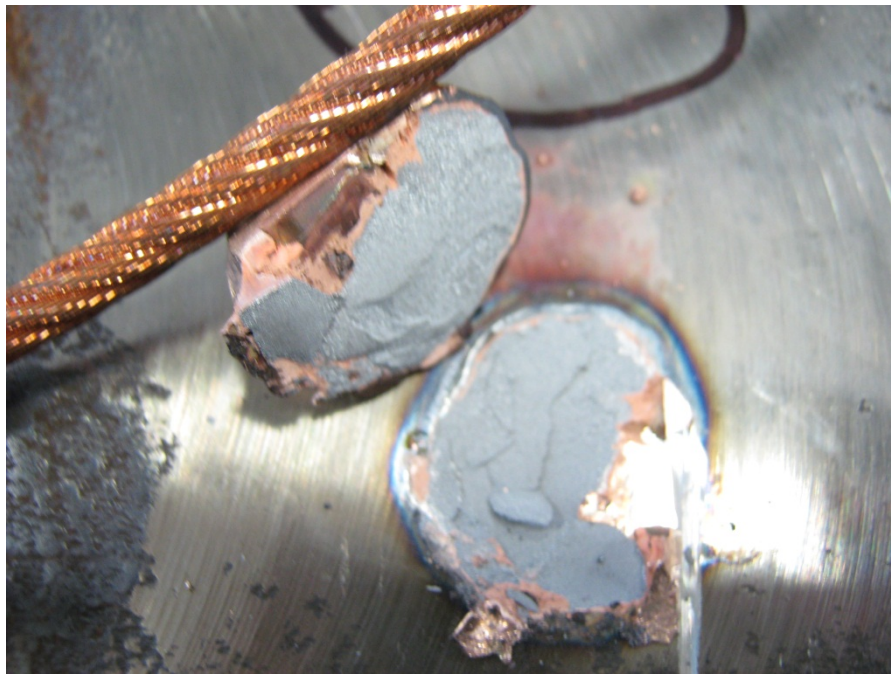
Figure 55. Fractured CAD Weld
