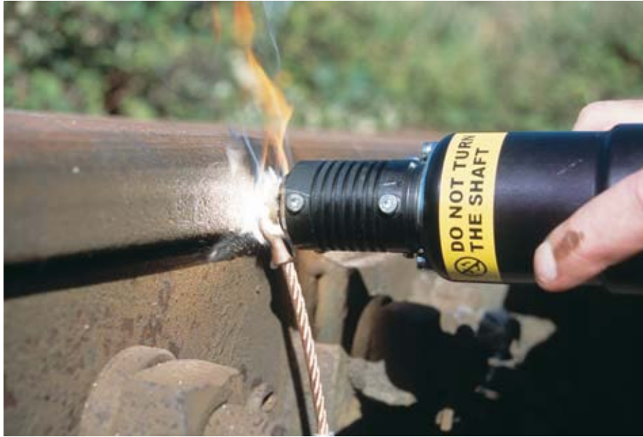
Figure 2. Pin Brazing
