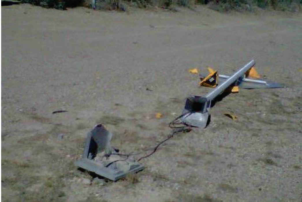
Figure 29. Stop Ahead Sign Knocked down a Week after Installation of the System.
