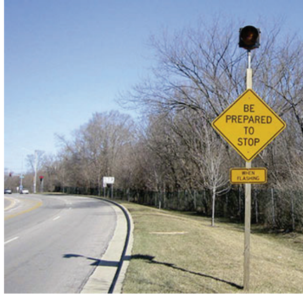
Figure 4. Example of Yellow Beacon on Advance Warning Stop Sign.
