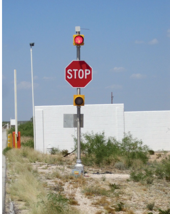
Figure 19. Stop Sign Installed at Pecos Test Track.
