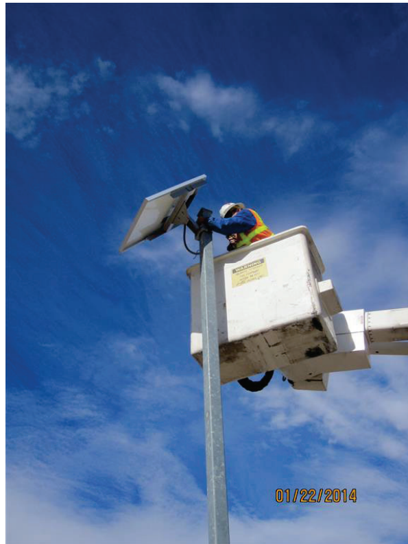
Figure 26. Access Point Installation on the Solar Panel Pole.
