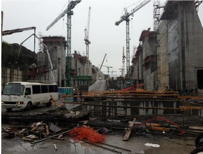
Figure 3 PCE under construction
