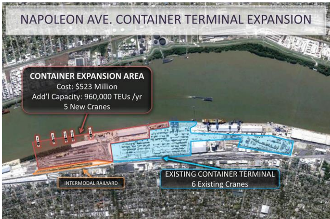
Figure 10 Napoleon Avenue Container Terminal Expansion
