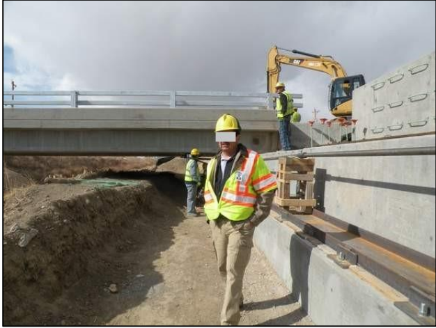
Figure 4.1 Fort Lyon Canal Bridge under construction
