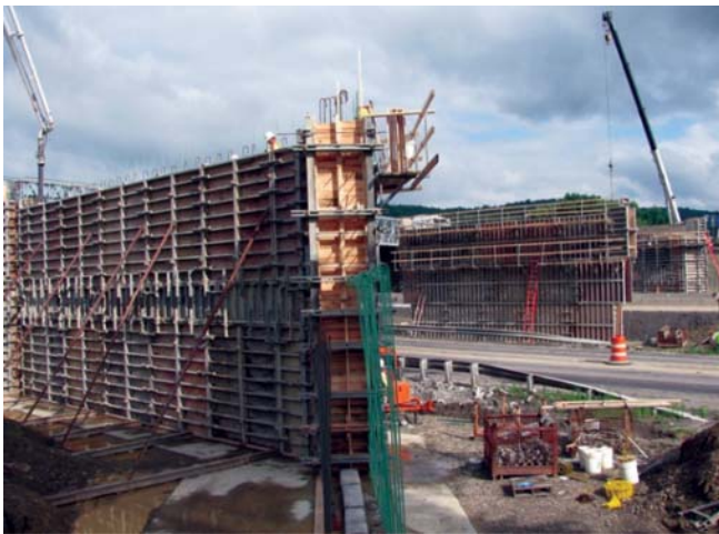
Figure 8. I-86 Coopers Plains bridge abutment stem structure in New York
