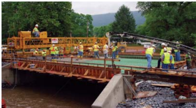
Figure 7. State Route 36, section 20, bridge deck in Pennsylvania
