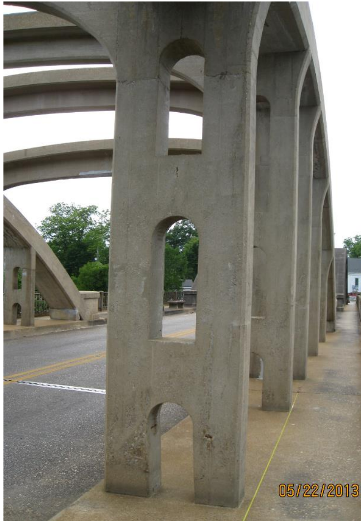
Figure 17: Concrete Hangers
