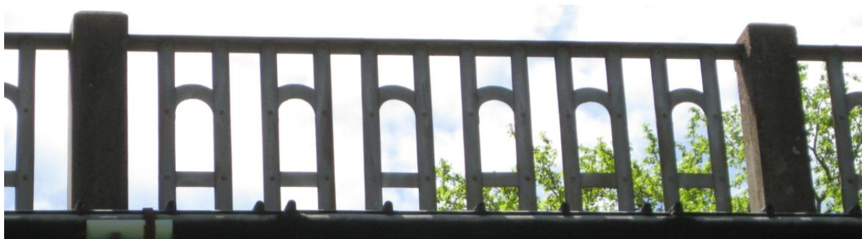
Figure 33: Side Railings on the Bridge
