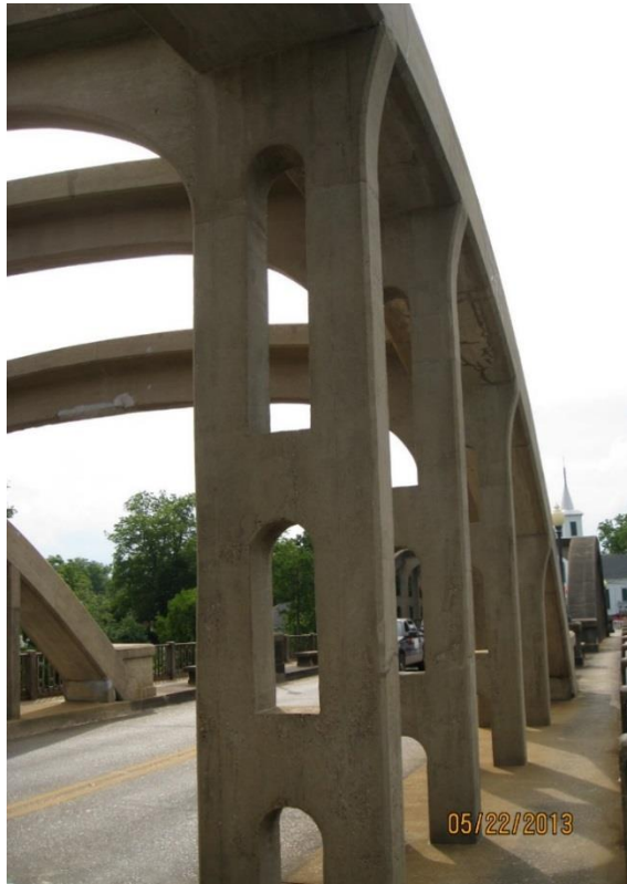
Figure 48: Composite Concrete Hangers
