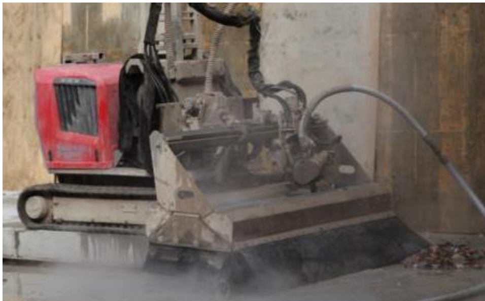
Figure 9. Hydrodemolition trial (Dang 2013)
