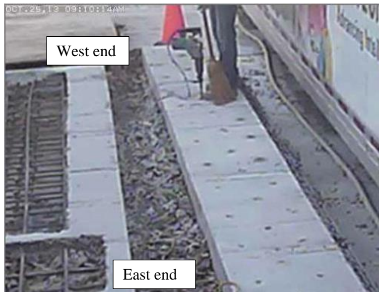
Figure 15. Drilling and cleaning holes taken by the networked camera
