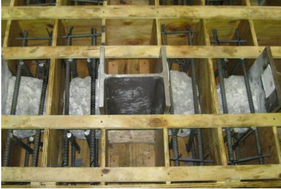
Figure 43. Specimens, reinforcing steel, and formwork (Dang 2013)
