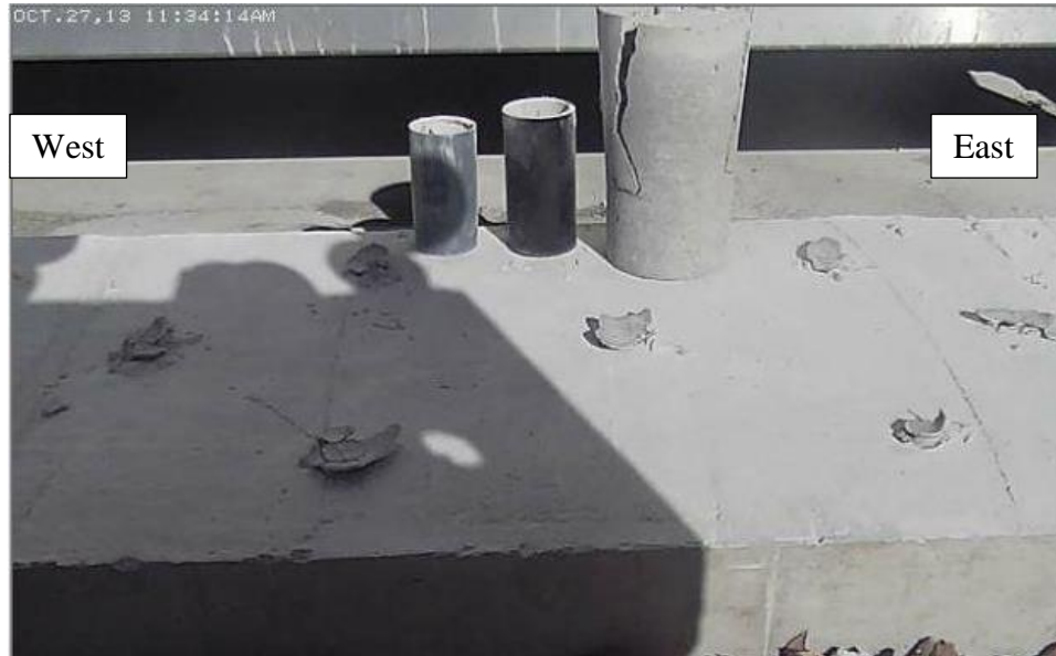
Figure 19. Chemical splitting on day two (after 48 hours)
