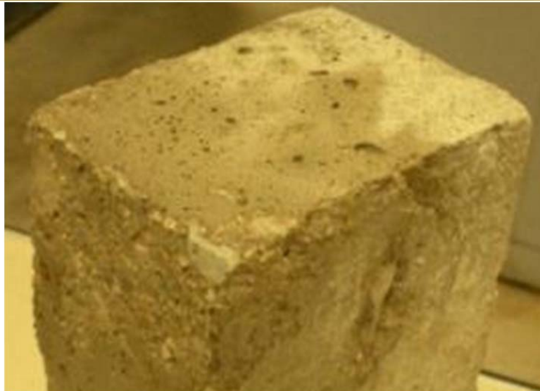
Figure O-34 Mix 13R–Specimen #4 (DF = 89.28, Fresh Air = 8%, Hardened Entrained Air = 9.08%)
