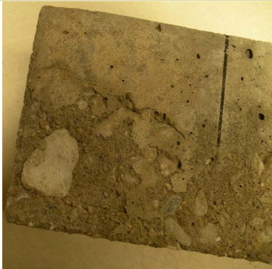
Figure O-9 Mix 1R–Specimen #3 (DF = 80.22, Fresh Air = 7.8%, Hardened Entrained Air = 8.04%)
