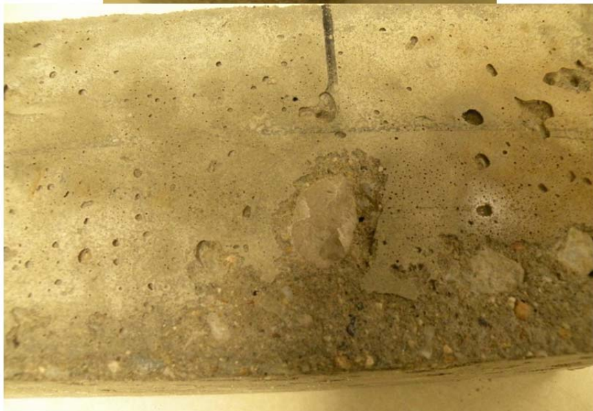
Figure O-8 Mix 1R—Specimen #2 (DF = 68.89, Fresh Air = 7.8%, Hardened Entrained Air = 8.04%)
