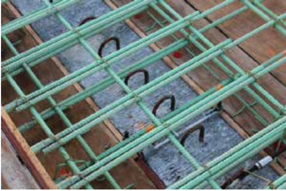
Figure 55. Rebar location and stirrup spacing on top of girder.
