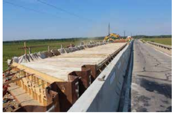
Figure 56. Southern half of bridge deck with cotton mat on top.
