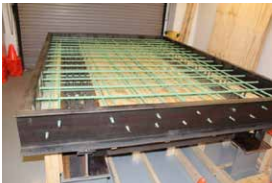
Figure 22. Deck with rebar and formwork.
