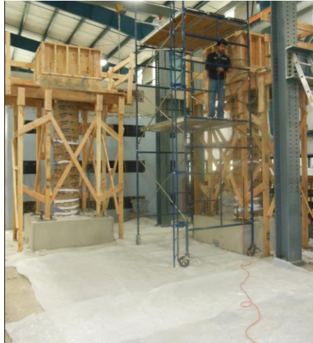
Figure 3.26 Photograph of the header and column formwork and shoring
