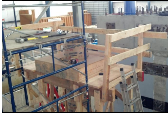
Figure 3.24 Photograph of the header shoring and false decking
