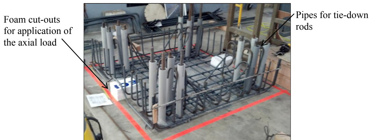
Figure 3.21 Photograph of Bottom reinforcing mat of the footing
