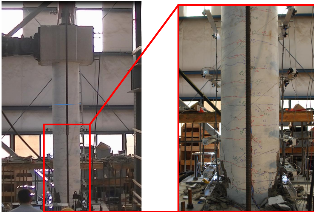
Figure 5.12 Column C2 crack mapping
