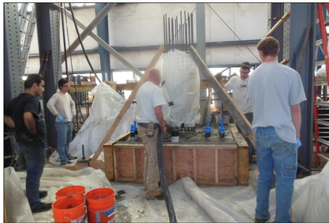
Figure 3.23 Photograph of the footing formwork and concrete pour
