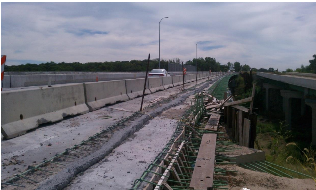
Figure 5.3 Completed Phase 1 under traffic load (September 14, 2013)
