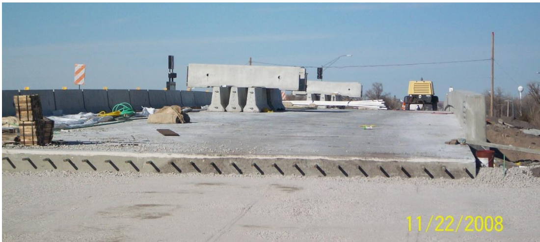
Figure 2.4: I-80 Hershey Interchange project in North Platte, NE after stacking barriers at the mid-span of second phase.
