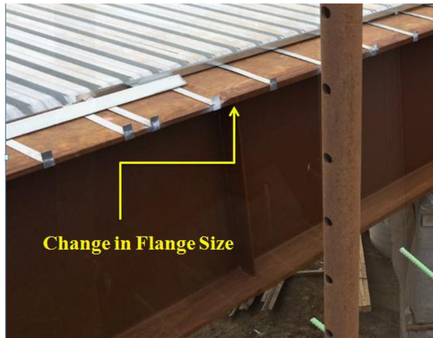
Figure 4.8: Plattsmouth Bridge Girder (February 28, 2014).
