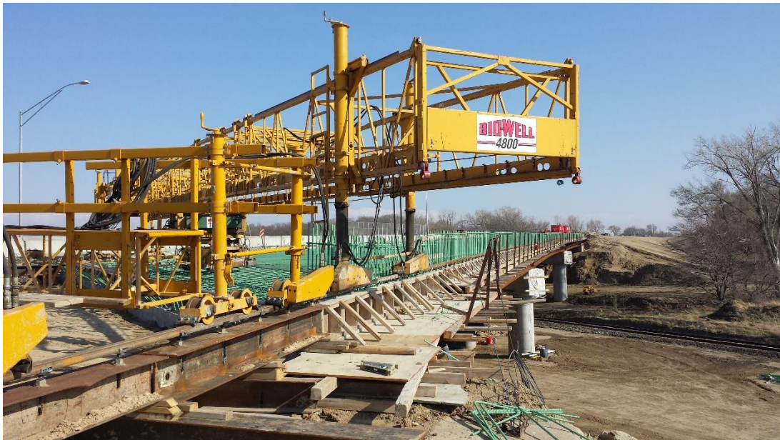
Figure 5.7 Preparation for Phase 2 deck pour (April 16, 2014)
