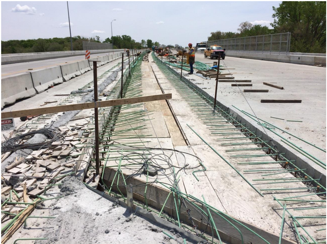
Figure 5.9 Phase 3 installed closure pour/ center median (May 14, 2014)
