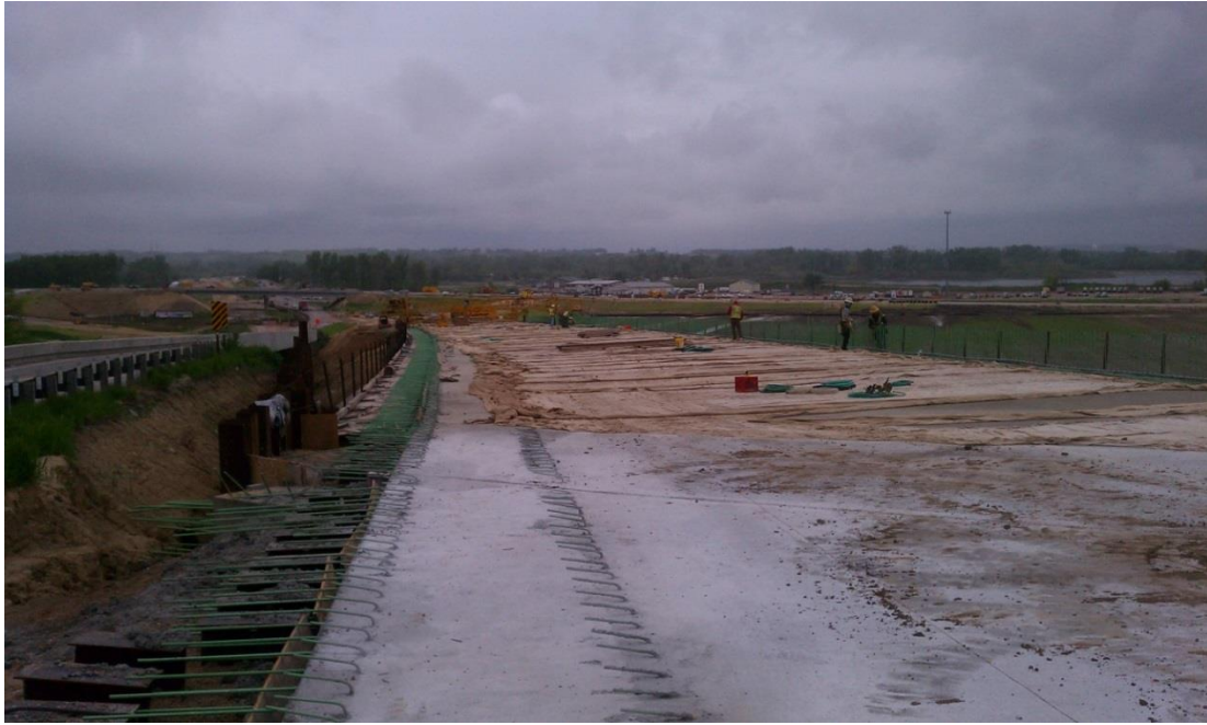
Figure 5.2 Phase 1 – Concrete Cure Process (May 22, 2013)
