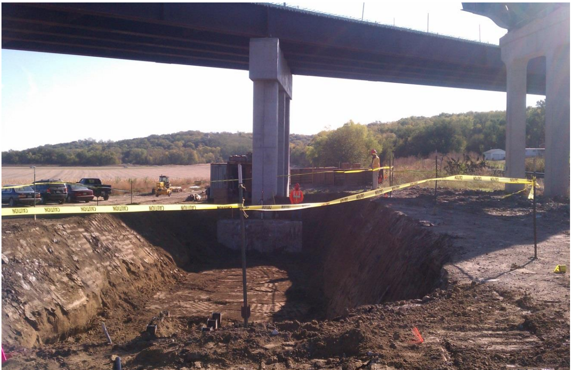
Figure 5.5 Phase 2 piers excavation
