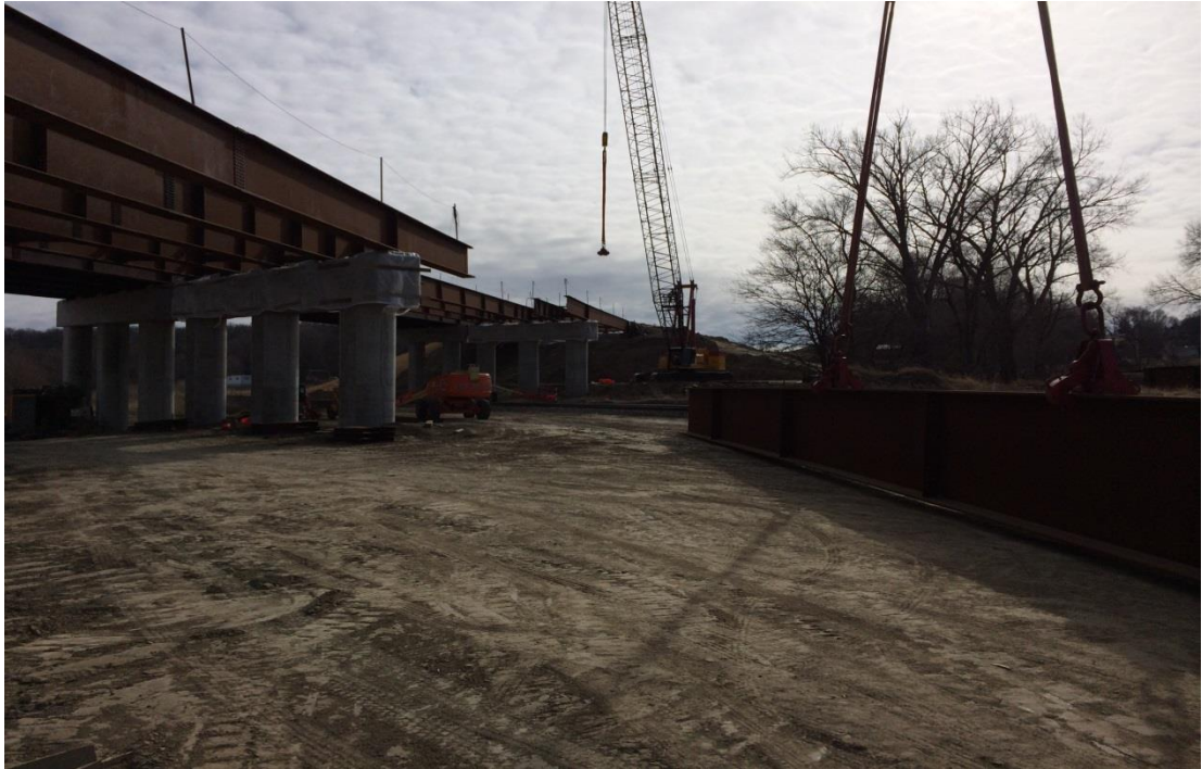
Figure 5.6 Setting of Phase 2 girders (January 24, 2014)
