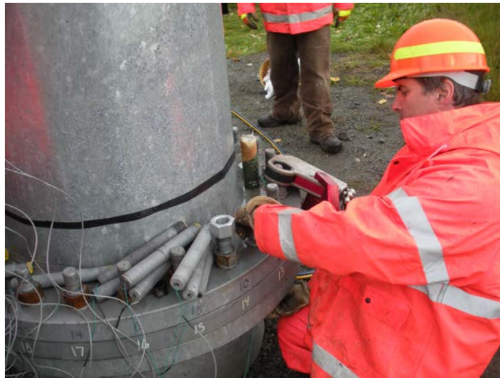
Figure 4.13: Installation and Tightening of Anchor Rods at Peter’s Creek HMLP
