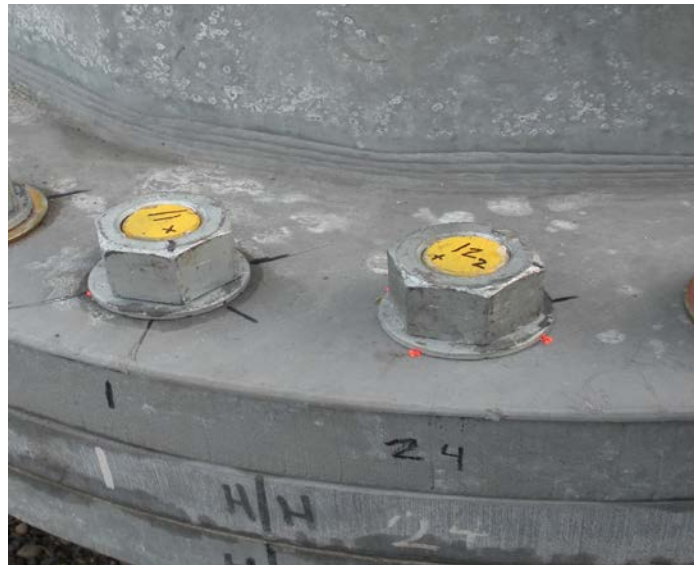
Figure 4.14: DTI Washers indicating full pre-tension during installation
