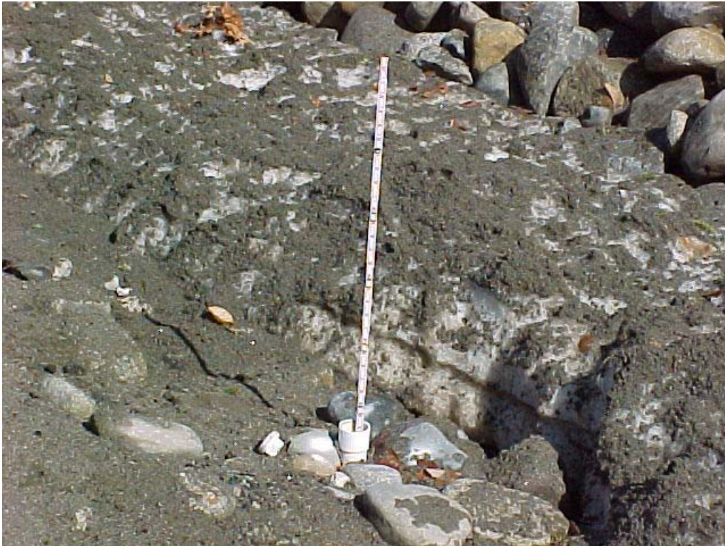
Figure 6. Measuring the Water Level in the Subsurface Drain
