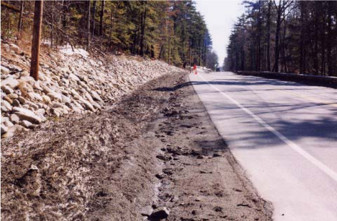
Figure 2. Ice & Snow Remain in the Ditch Long After Other Areas Have Melted
