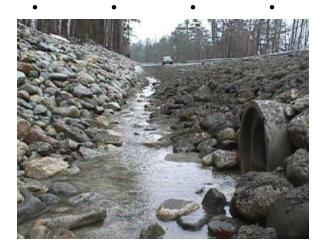
Experimental Construction Report ME 00-20 First Year Interim Report on Experimental Utilization of Tire Shreds to Enhance Highway Drainage June 2001
