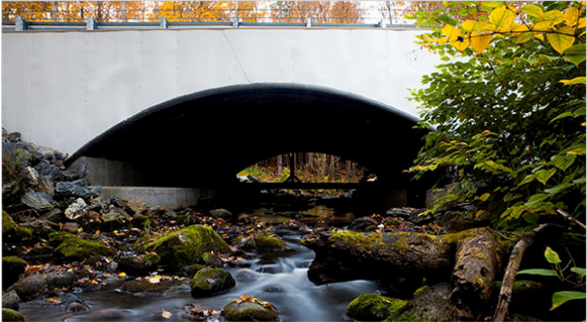
Figure 4.16 Bridge Demonstrating End Arch Exposure to Sunlight
