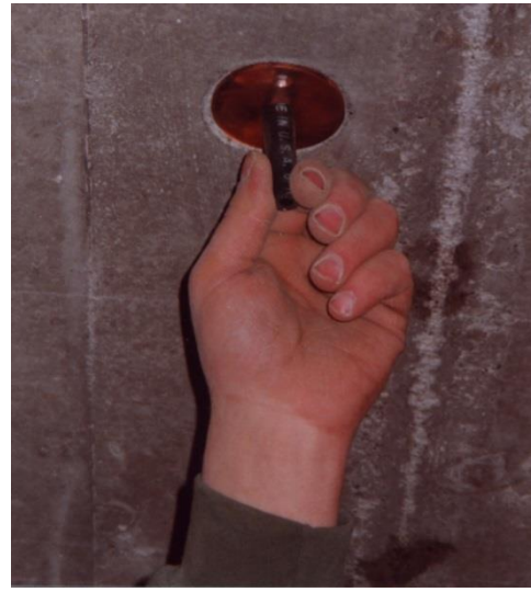
Figure 4.2b: Epoxy Primary in Place
