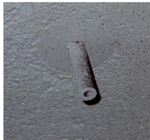
Figure 4.2d: Apply TS Zinc
