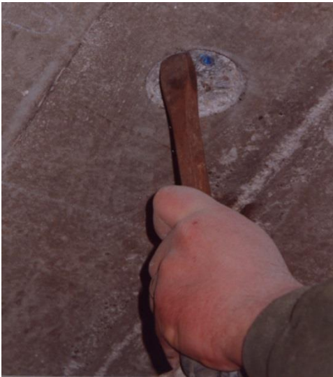
FIGURE 4.2a: Cut Recess for Primary
