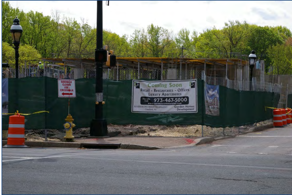
Figure 30. Riverfront at Cranford Station, under construction (Spring 2012)
