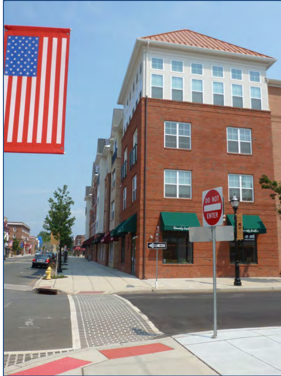
Figure 52. Park Square, Rahway, NJ
