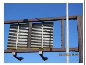
No deficiencies of the horizontal chords and secondary vertical posts were found. This element was rated as 1 (Structure #01-20-64-57.88 - type 1.1).
