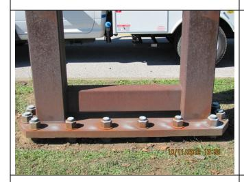
No deficiencies of the weld lines between the column vertical members and the supplemental bracing were found. This element was rated as 1 (Structure #01-20-60-11.44 - type 3.3.1).
