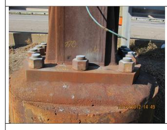
No deficiencies of the anchor bolts, nuts, and washers were found. This element was rated as 1 (Structure #01-20-77-101.24 - type 1.1).
