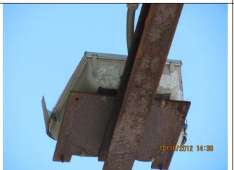
Minor to moderate corrosion of the lower chord was observed. This element was rated as 3 (Structure #01-20-77-102.49 - type 1.1).
