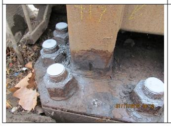
Minor to moderate corrosion of weld lines 1 and 2 connected between the base plate and the median vertical column was observed. This element was rated as 3 (Structure #01-20-79-01.12 - type 4).
