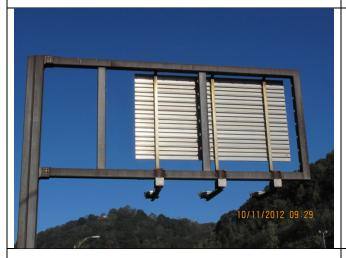
No deficiencies of the attachments were found. This element was rated as 1 (Structure #01-20-77-97.32 - type 1.1).
