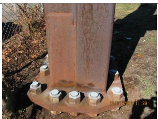
Minor corrosion of weld line 1 connected between the base plate and the vertical column was observed. Weld reinforcement had been starting to deteriorate. This element was rated as 2 (Structure #01-20-77-97.32 - type 1.1).
