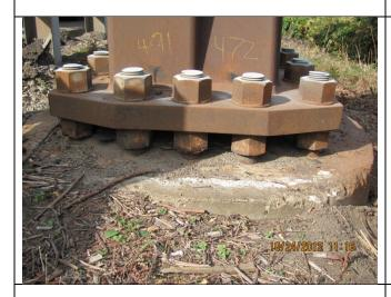
No grout pad was present under the base plate. This element was rated as 1 (Structure #01-20-64-55.85 - type 1.1).
