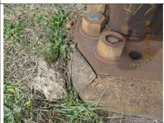
Mortar cracking of the grout pad under the base plate at the left vertical column was observed. This element was rated as 2 (Structure #01-20-77-101.23 - type 3.1).
