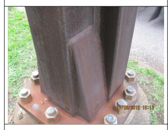
No deficiencies of the connection between the base plate and the vertical column were found. This element was rated as 1 (Structure #01-20-64-52.40 - type 1.1).
