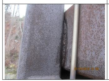
Pack rust between plates/members was observed. One U-bolt connected the shoulder vertical column and the upper chord was loose. This element was rated as 3 (Structure #01-20-64-57.53 - type 4).
