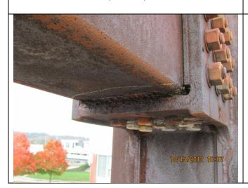
Minor corrosion of bolts connected between the vertical column and the lower chord was observed. Severe pack rust between plates/members in the lower chord was reported. One bolt was completely loose and the rest were somewhat loose. This element was rated as 4 (Structure #01-20-64-57.83 - type 1.1).
