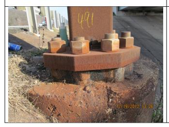
Concrete spalling of the foundation under the left vertical column was observed. This element was rated as 2 (Structure #01-20-77-100.98 - type 3.1).
