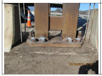
Minor section loss and surface pitting of the base plate on the median vertical column was reported. Minor to moderate corrosion of the base plate was observed. This element was rated as 3 (Structure #01-20-64-58.30 - type 5).
