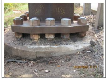
Minor to moderate corrosion and deterioration of leveling nuts/washers was observed. This element was rated as 3 (Structure #01-20-64-55.85 - type 1.1).
