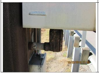
Minor corrosion of horizontal light arms was observed. Pack rust between light arm JB's and the lower chord was reported. LB from the electrical box was corroded. This element was rated as 3 (Structure #01-20-64-55.12 - type 1.1).
