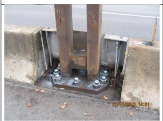
Corrosion on bottom of the weld lines connected between the median vertical column and the supplemental bracing was observed. This element was rated as 2 (Structure #01-20-64-57.52 - type 4).
