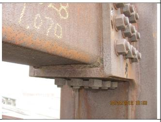
Minor corrosion of bolts connected between the lower chord and the vertical column was observed. Pack rust between plates/members was reported. This element was rated as 2 (Structure #01-20-64-55.85 - type 1.1).
