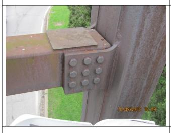
No deficiencies of the connections between the vertical column and the horizontal chord were found. This element was rated as 1 (Structure #01-20-64-52.40 - type 1.1).
