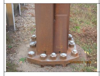
No deficiencies were found in the base plate. This element was rated as 1 (Structure #01-20-64-56.50 - type 1.1).
