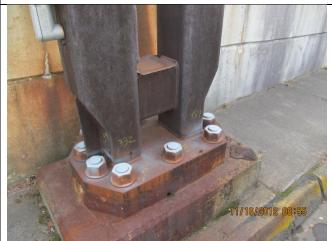
Minor corrosion of the base plates on the left/right vertical columns was observed. This element was rated as 2 (Structure #01-20-77-100.08 - type 3.2).
