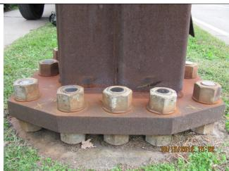
Two anchor bolts were slightly cut short. Minor corrosion of two anchor bolts and leveling nuts/washers was observed. This element was rated as 2 (Structure #01-20-64-57.83 - type 1.1).
