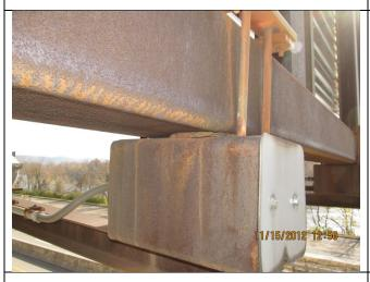
Minor corrosion of horizontal light arms and vertical sign support to horizontal chord connection bracket was observed. Pack rust between light arm JB's and the lower chord was reported. This element was rated as 2 (Structure #01-20-77-97.95 - type 1.1).
