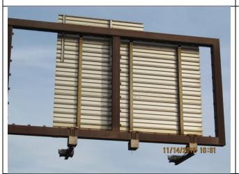
Minor corrosion of horizontal chords and secondary vertical posts was observed. This element was rated as 2 (Structure #01-20-64-58.54 - type 1.1).
