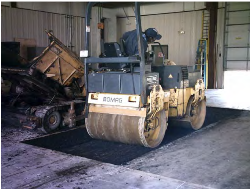
FIGURE 2.8: Compaction of Asphalt Concrete
