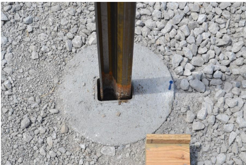
Figure 12. Fabrication and Installation Photographs
