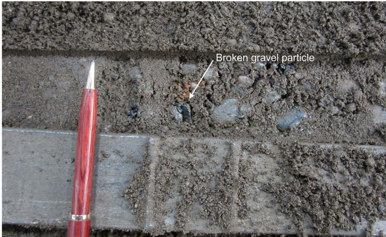
Figure 0.11 Photo of a gravel particle crushed by a reinforcement rib.
