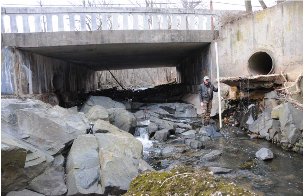
Photo 3.2. Bed degradation into fractured bedrock at the Strathmore Avenue Bridge over Western Run, Baltimore City.
