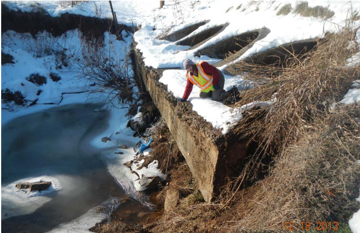
Photo 3.1. LTBD measured at culvert apron of Gas House Pike, Frederick County.
