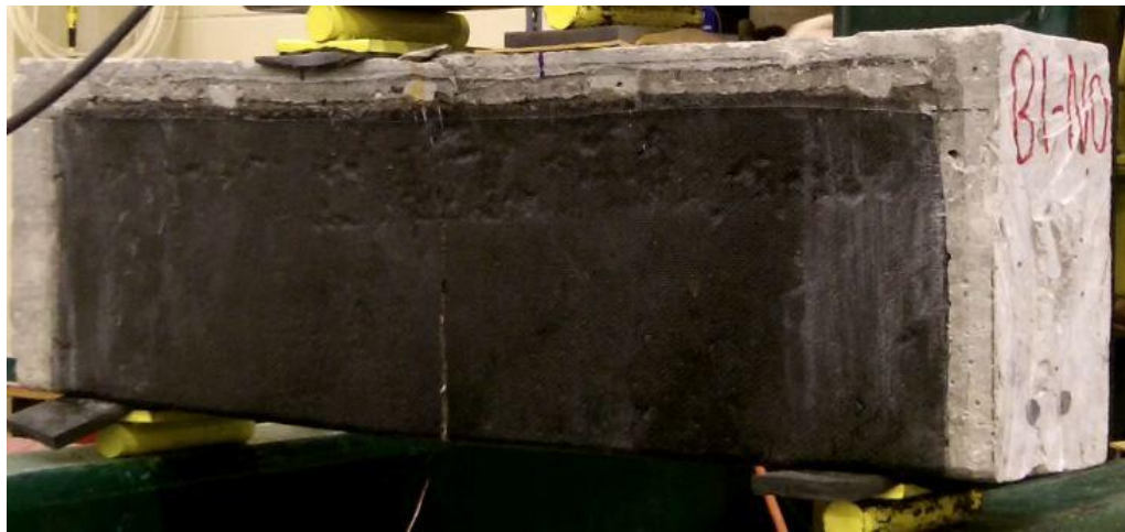
Figure 10: 279 mm Deep Beam, B1, No Grooves, after Failure
