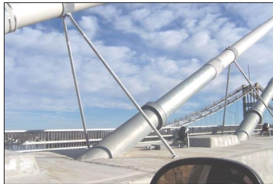
Figure 38. Photo. Damper's attachment to cable and median slab.
