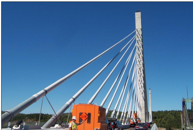
Figure 14. Photo. Bridge cable fan configuration.
