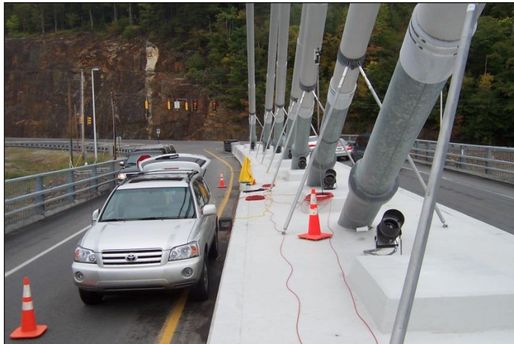
Figure 16. Photo. Detail of lower end of bridge cables.
