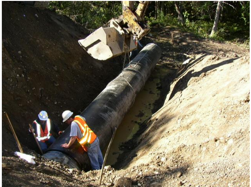
Figure 4 Placing inlet half of overflow pipe in Benedicta.
