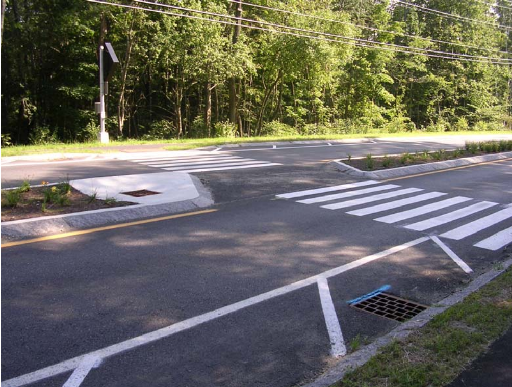
Figure 14 Detail of crosswalk area with drainage grates
