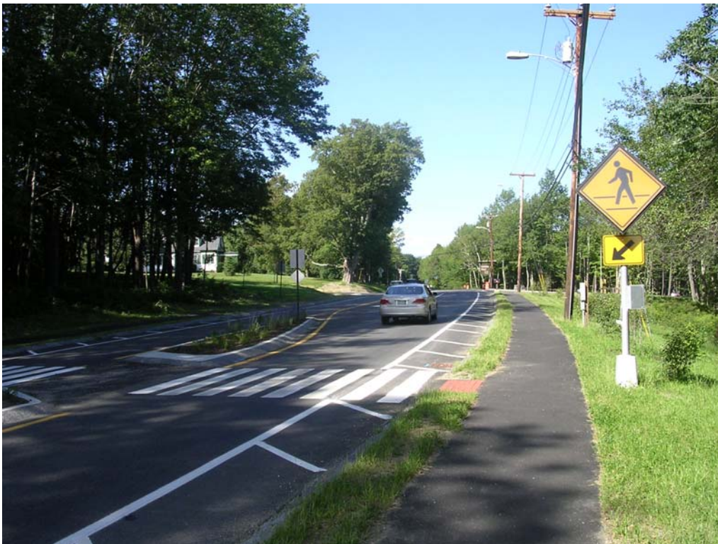
Figure 13 Crosswalk with flashing sign activated by pedestrian push button
