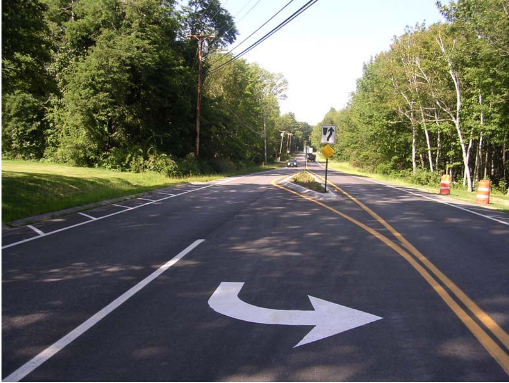
Figure 10 Looking northbound at northern refuge island
