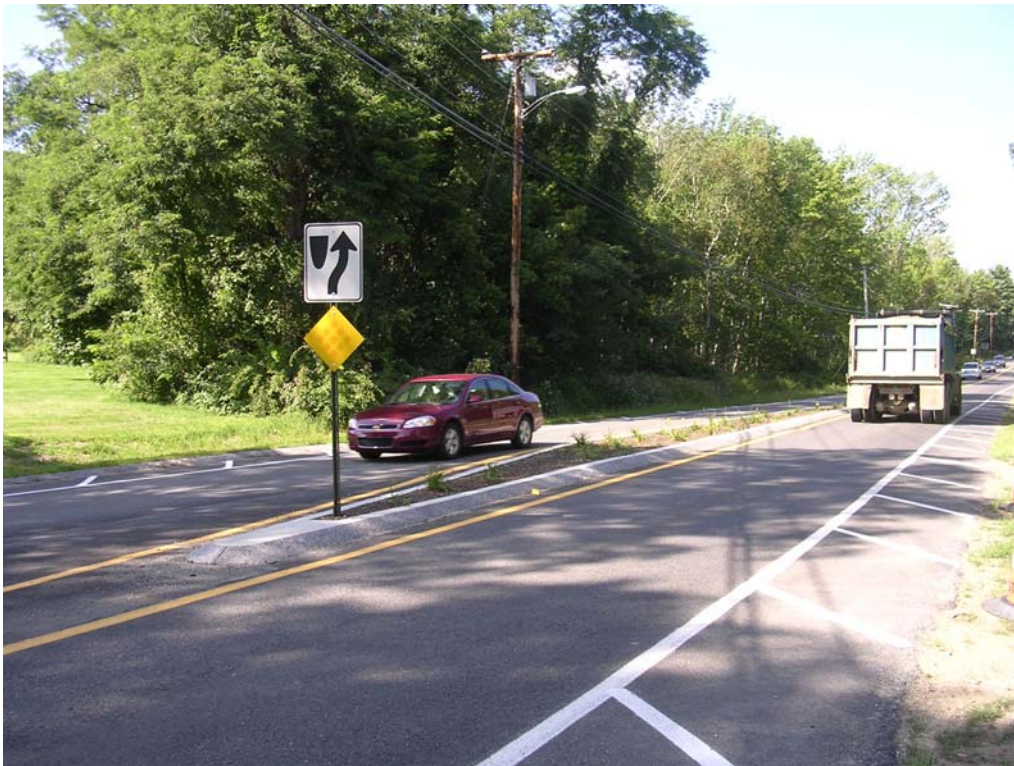
Figure 11 Looking northbound at the northern refuge island, showing 'narrow' lane
