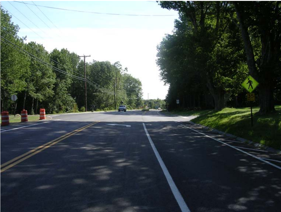
Figure 9 Southbound left-turn lane photographed just south of Figure 8
