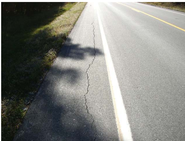
Photo 2: Shoulder Crack – 2007
