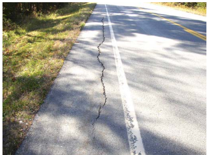
Photo 3: Shoulder Crack – 2008
