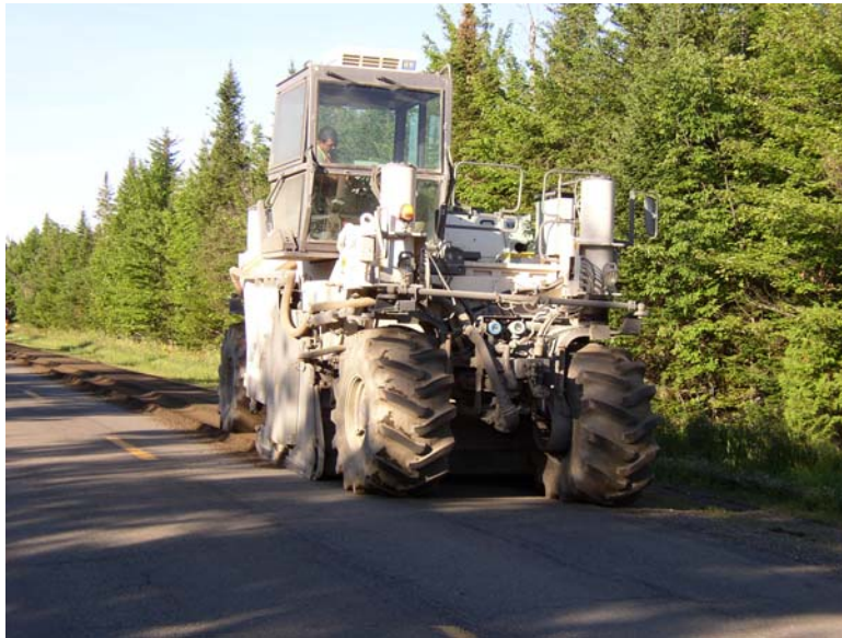
Photo 2: First Pass with the Wirtgen 2500 Recycler
