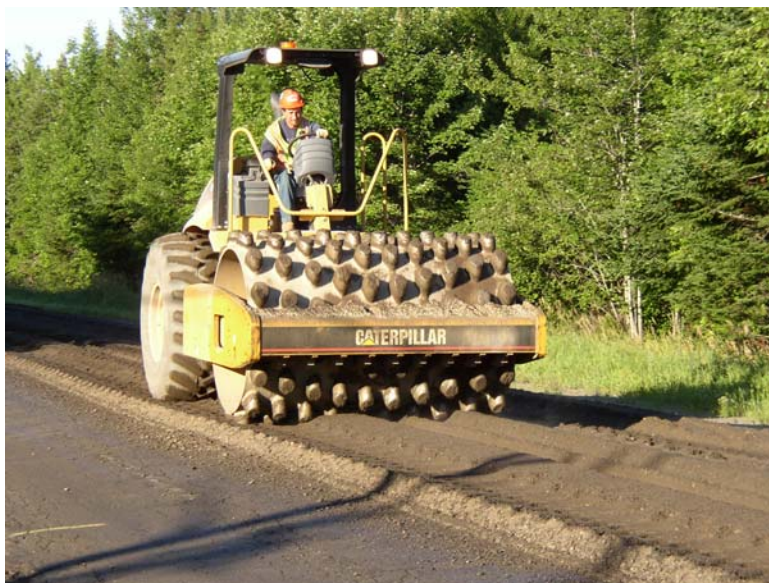
Photo 3: Pad Foot Vibratory Roller
