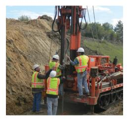
Researchers installed sensors by pushing them into the ground with a common drill rig.
