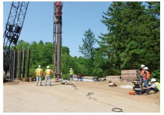
Researchers used sensors (shown in foreground, connected via cables) to measure vibrations at various distances from pile driving operations, both on the surface and at various depths.
