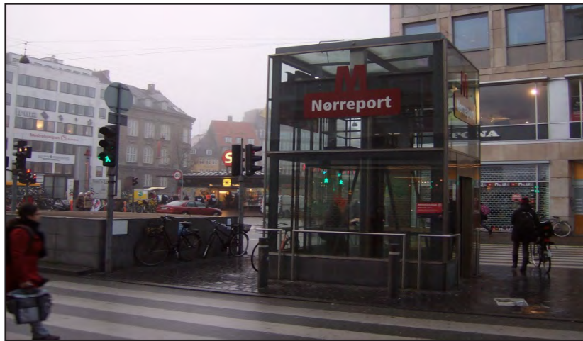
Figure 60. Copenhagen Driverless Metro
