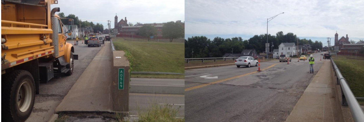
Figure 2-1 Bridge A0569 Overview of Bridge Deck Observed During Field Investigation
