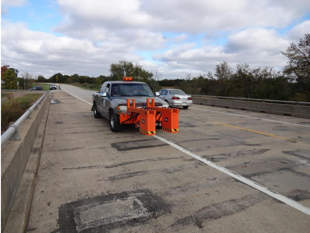
Figure 2-3 Bridge A3406 Overview of Bridge Deck Observed During Field Investigation
