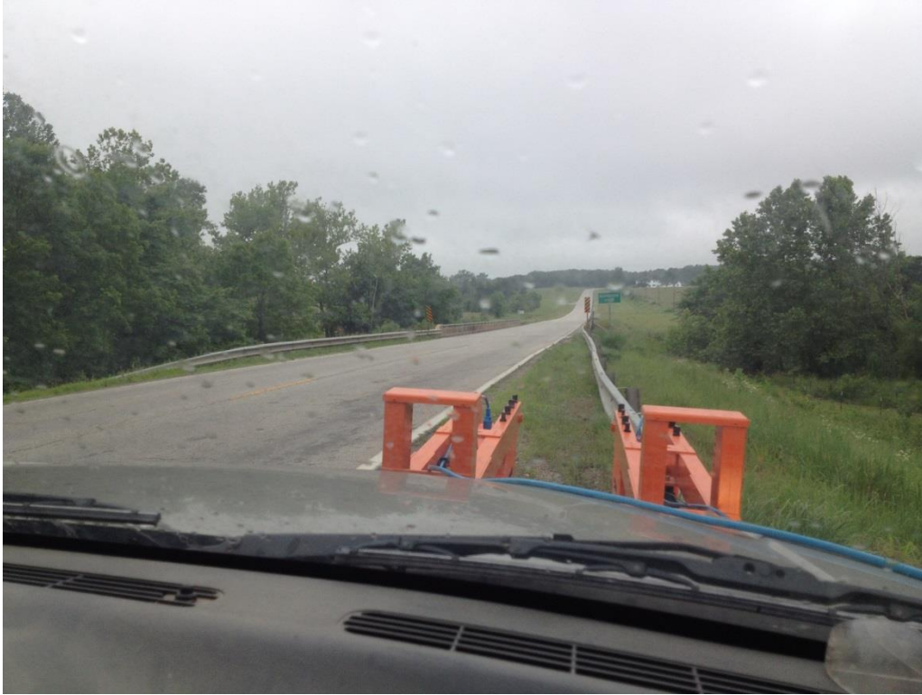
Figure 2-6 Bridge K0197 Overview of Bridge Deck Observed During Field Investigation
