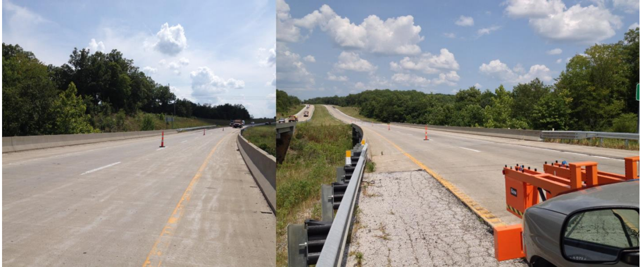
Figure 2-4 Bridge A4780 Overview of Bridge Deck Observed During Field Investigation
