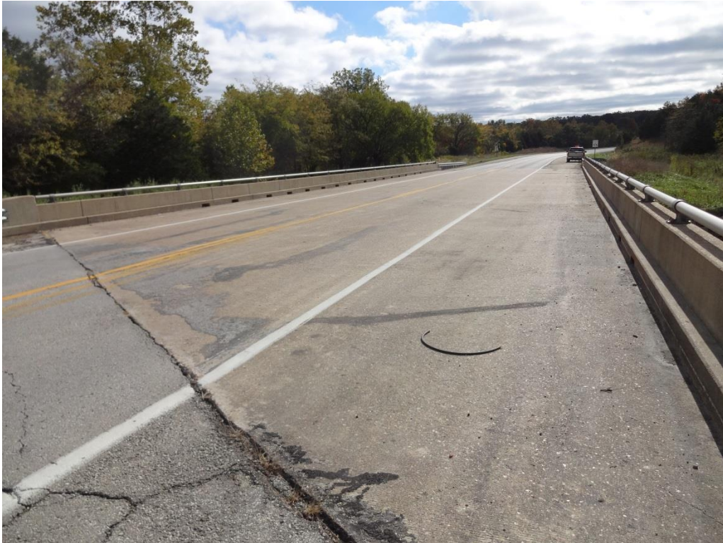
Figure 2-2 Bridge A3405 Overview of Bridge Deck Observed During Field Investigation
