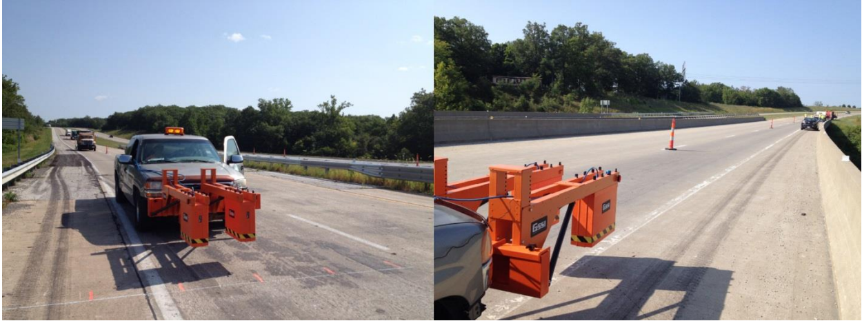
Figure 2-5 Bridge A4781 Overview of Bridge Deck Observed During Field Investigation
