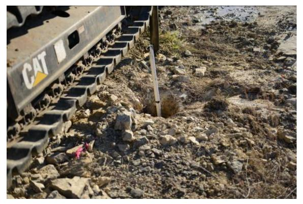
Figure 6: Piezometer installation.
