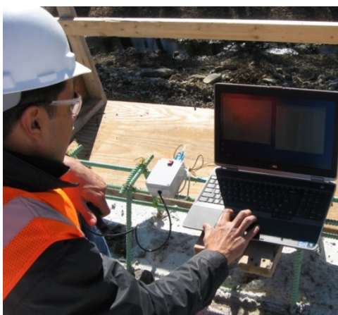
Figure 3.1. Bridge A7957 Data Acquisition
