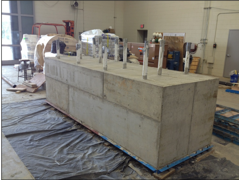
Figure (9): Reinforced Concrete pedestal
