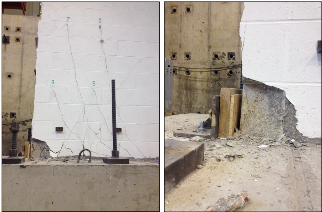
Figure (36): The toe failure for wall 1
