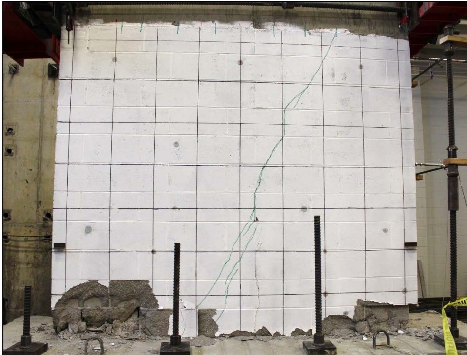
Figure (41): The general failure of wall 2
