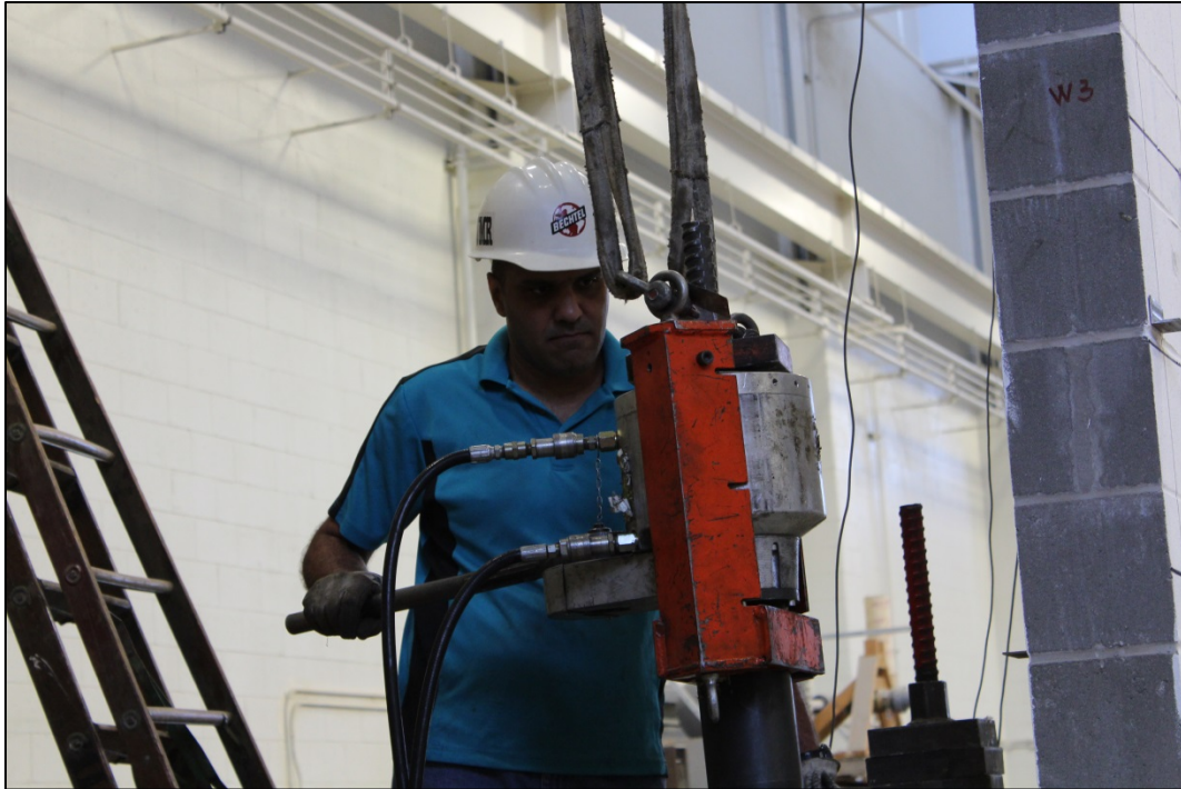
Figure (19): Applying the post-tensioned forces by using hydraulic jack
