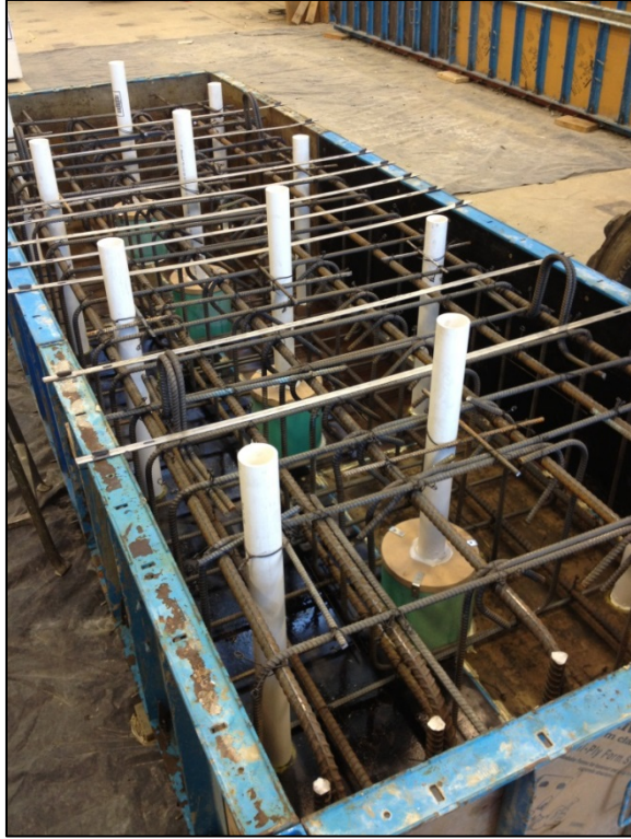
Figure (8): Reinforcements and holes in wall footing
